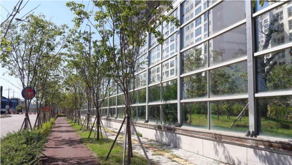
Figure 2. An example of transparent noise barriers (TNB) that may cause bird collisions
